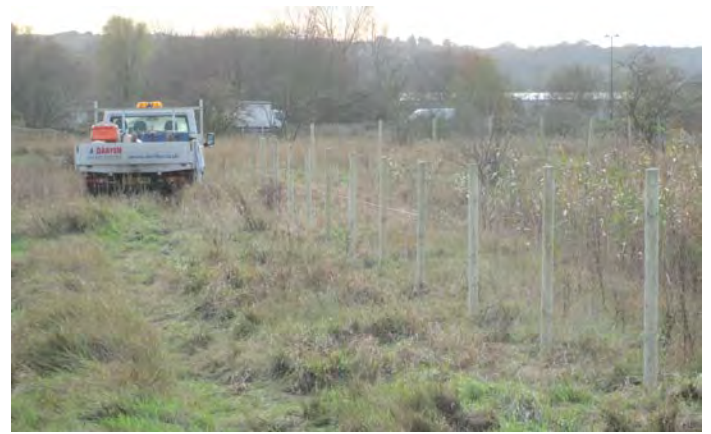
Post and wire fencing alongside Great Breach Lagoon
