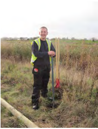
Kev digging holes for the posts
