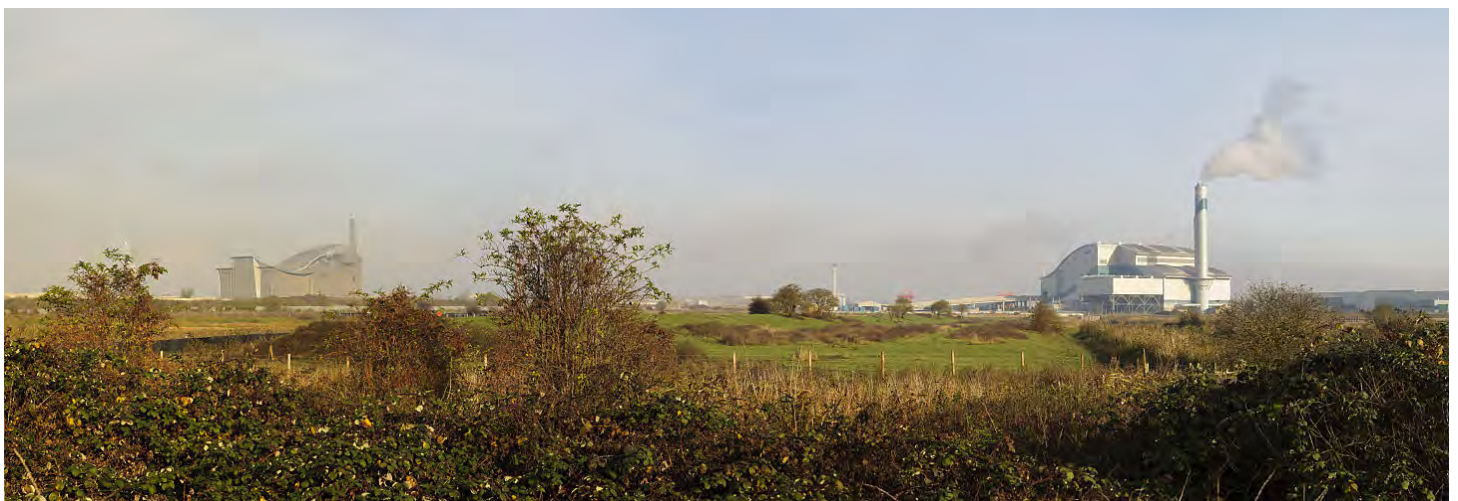
Beautiful photo of the nature reserve (looking north from Footpath 1), Thames Water's Crossness Sludge Powered Generator (left) and Cory Environmental's Riverside Resource Recovery facility (right). Photo by David Pressland, used with kind permission
