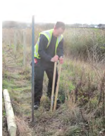
Putting post hole digger to use
