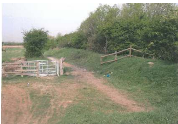
Damaged fencing and extensive motorbike tracks
