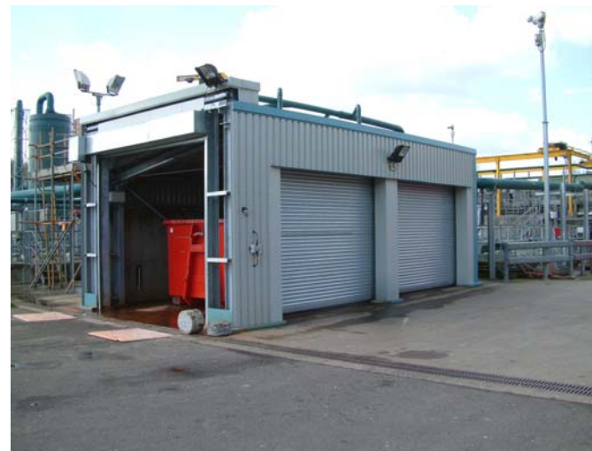
Grit Skip Enclosure (West)
