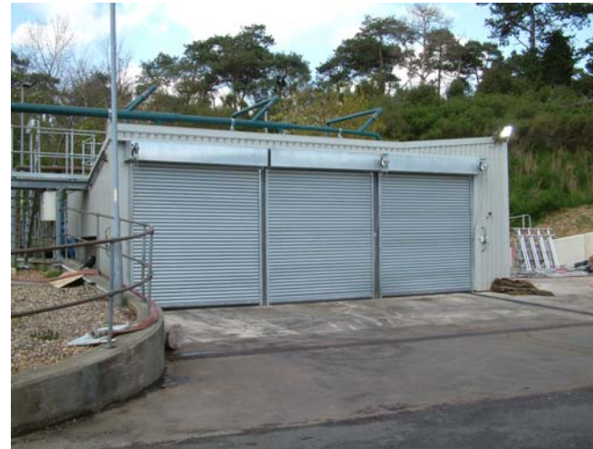
Grit Skip Enclosure (East)
