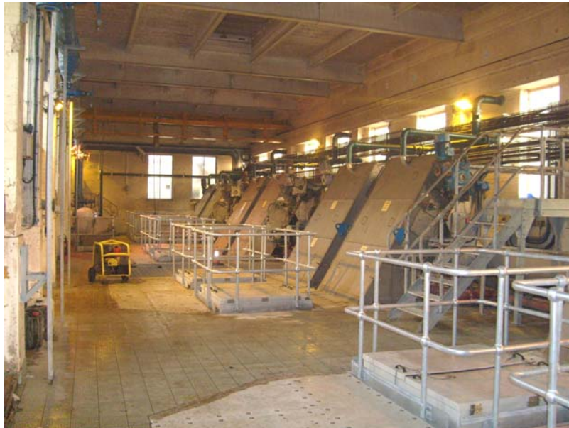
Screen House (East)
