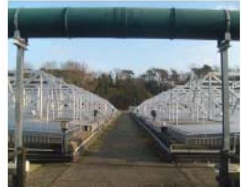
Storm Tanks 4 & 5 (East)
