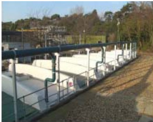
Storm Weir (East)
