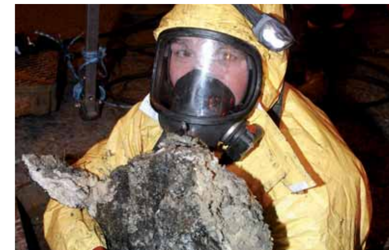
Contractor removing fat from sewer wall
