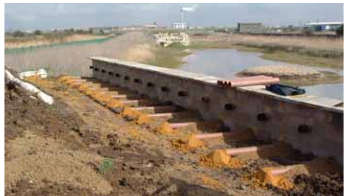
The back of the sand martin bank during construction
