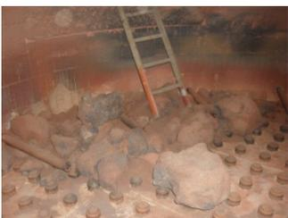
**Inside Beckton Sludge Powered Generator during refurbishment**
