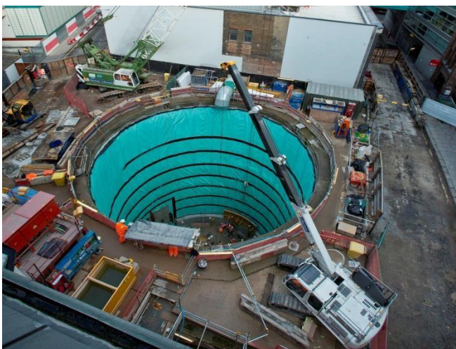
Deep excavation using heavy machinery
