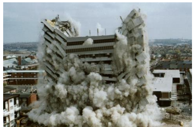
Demolition using explosives
