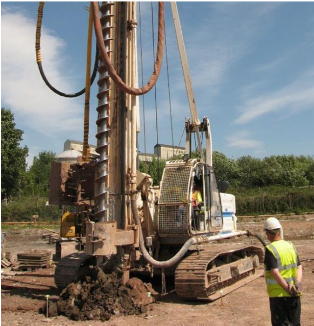
Continuous flight auger method of piling
