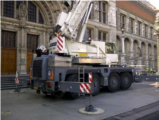
Crane positioned on riggers, transferring loading to the ground
