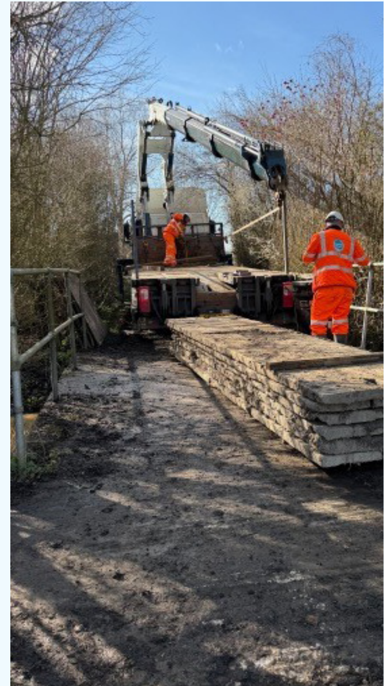
The bridge to the field where the burst was located
