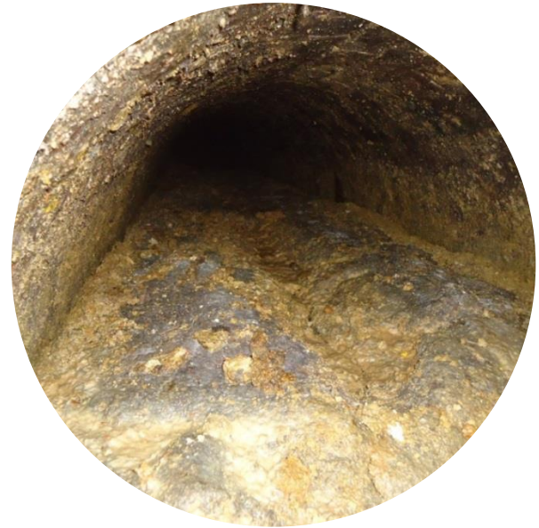
FOG blocking our sewer pipes which can lead to flooding and pollution to homes, businesses and the environment.
