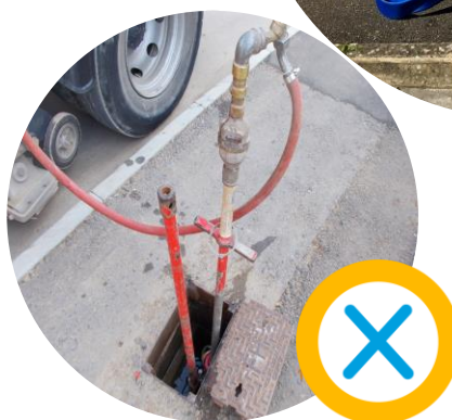
Thames Water authorised standpipes (above) and an illegal connection (left)
