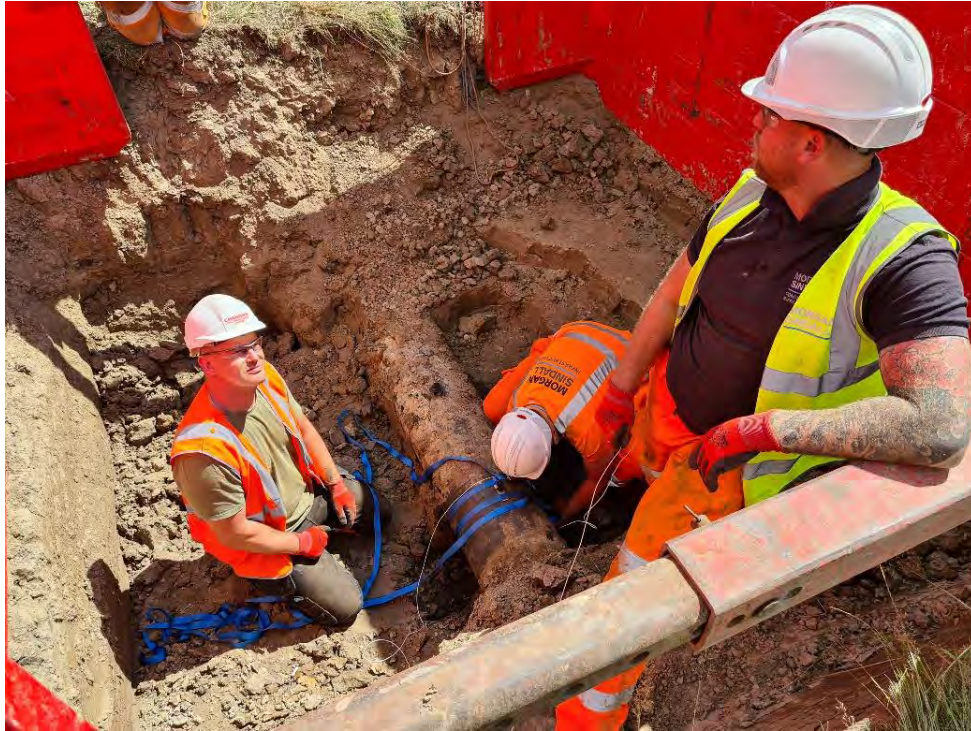
Accelerometer installation on the pipe
