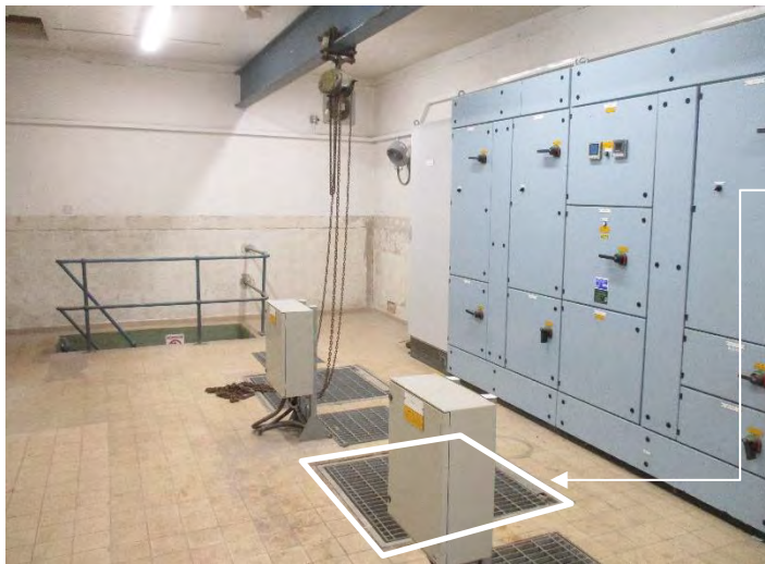
Figures 8a & 8b Control room & equipment hoist access (highlighted)
