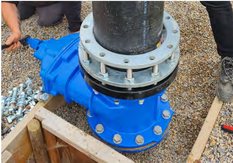
Figure 6 DN300 Gate valve on vertical flange of equal tee, launch tube attached.
