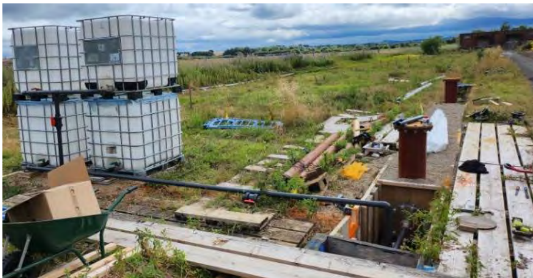
Figure 3 Test rig connected to stacked water IBCs via 2" pipework
