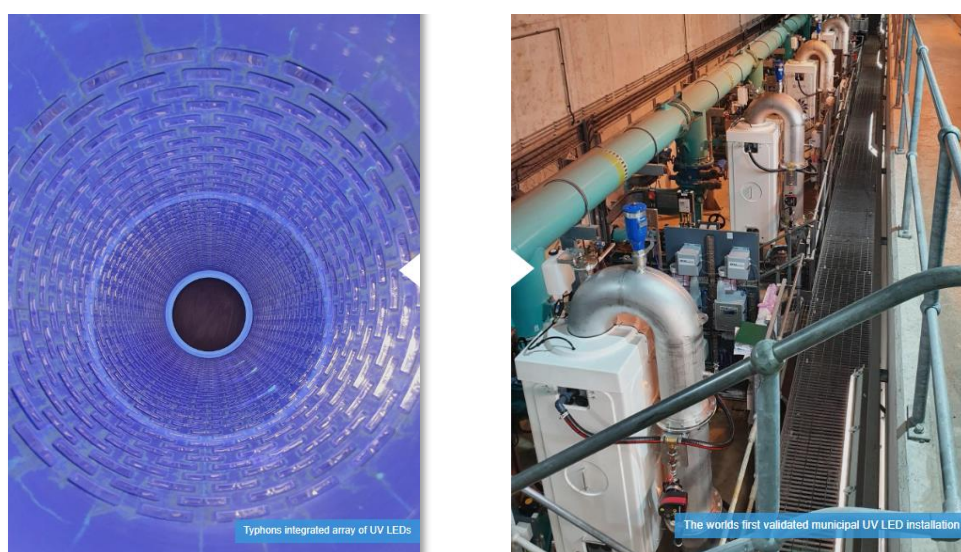
Figure 10.2 UV LED technology deployed to inactivate Cryptosporidium – see footnote 58
