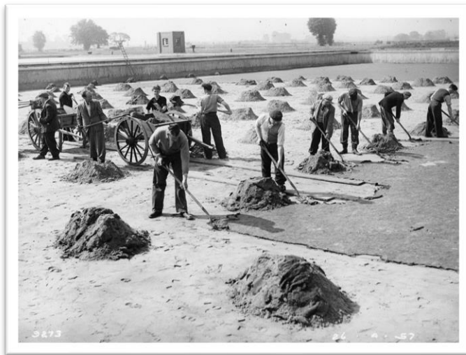
Figure 9.1: Labour intensive SSF cleaning well in to the 1950s at Hampton WTW
