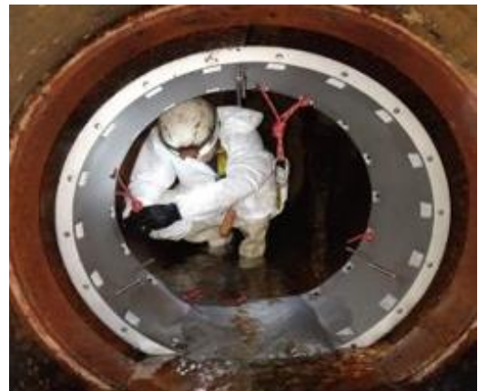
Our team reinforcing joints on existing pipework
