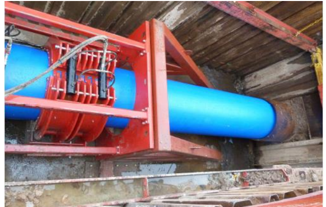
Inserting plastic pipe into the old iron water main.
