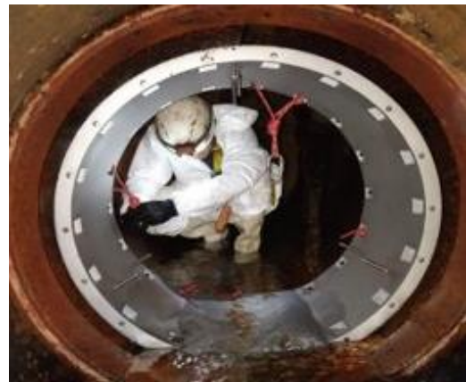
Our team reinforcing joints on existing pipework
