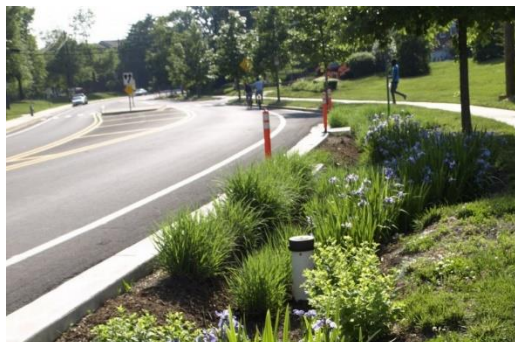
Figure 1.1: SuDS features installed as part of CCFAS
