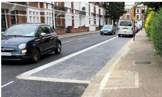
Figure 1.1: SuDS features installed as part of CCFAS
