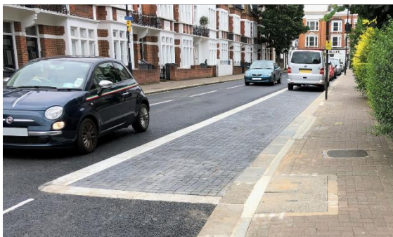
Figure 3.1: SuDS features installed as part of CCFAS
