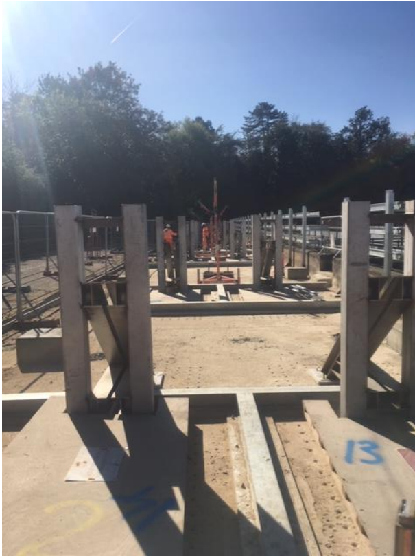
Aerator Guide Rails
