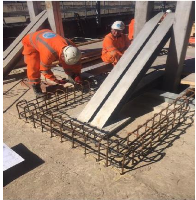
Aerator Upstand Construction
