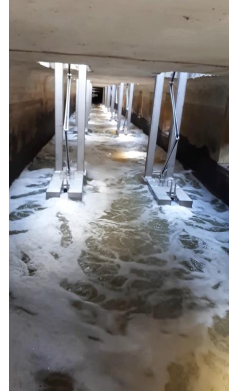
Floating Aerators in action
