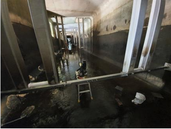
Guiderrail restraint install
