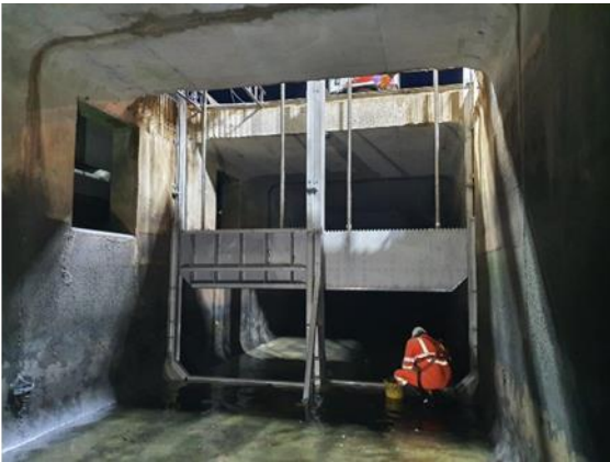
Weir penstock install
