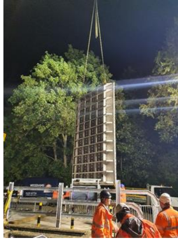
Stopgate being lifted into place for isolation
