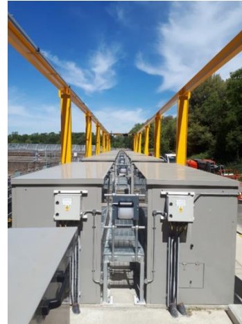
Aerator Kiosks with view of overhead crane
