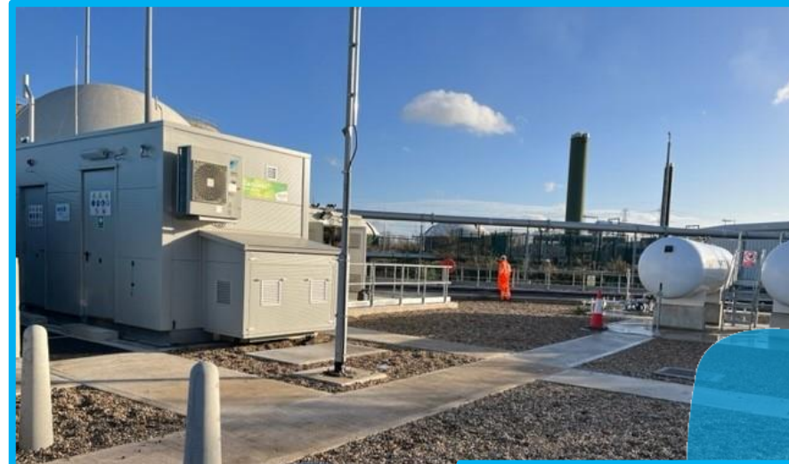
View of compressor plant and propane dosing tanks
