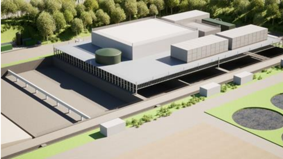
Photomontage of the TTP at Mogden STW, located on a platform over the existing storm tanks
