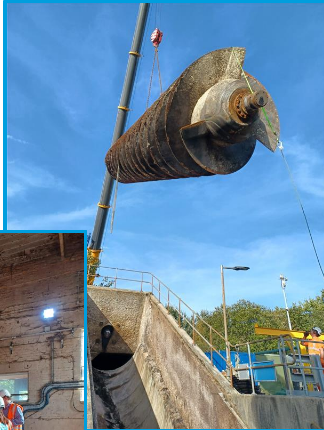
Screw Pump No. 1 Remedial works
