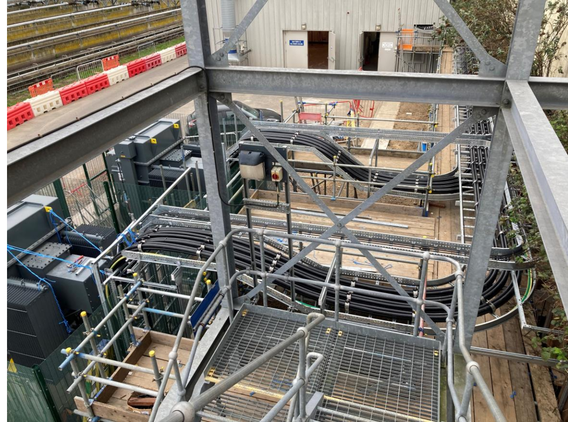
Battery E New Transformers Cabling to MCC
