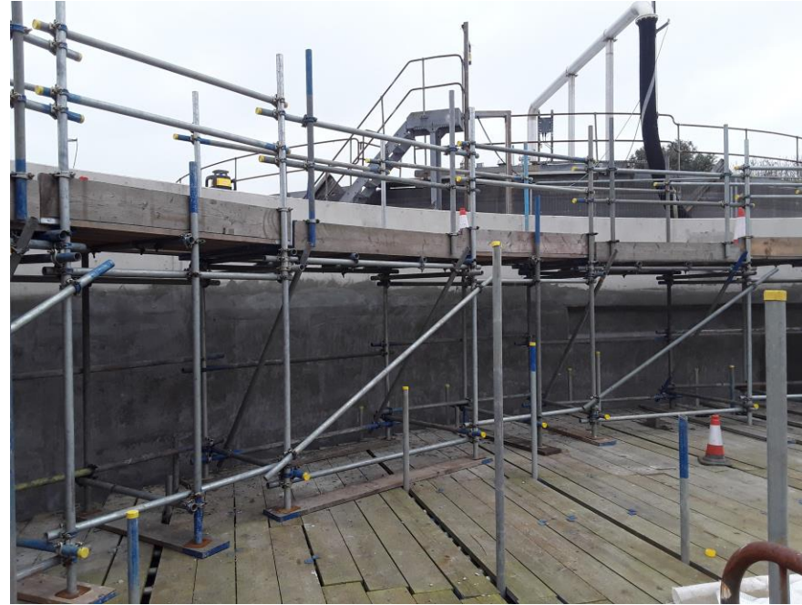
Digester 16 – Coating Complete
