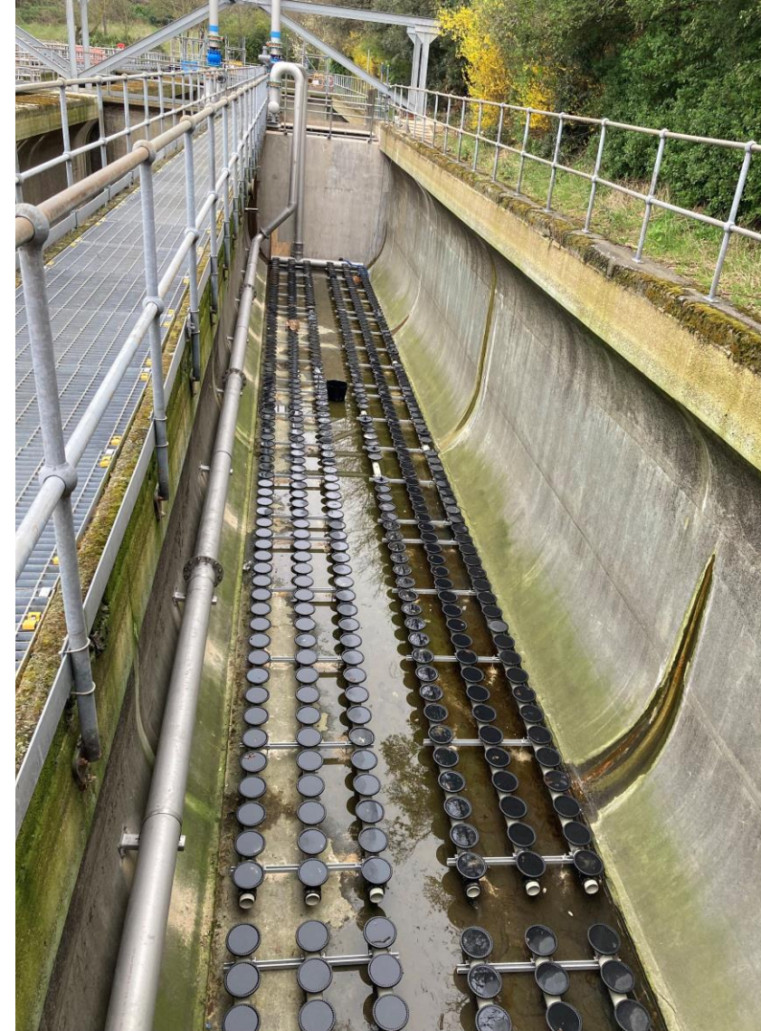
Lane 13 Diffuser Pipework
