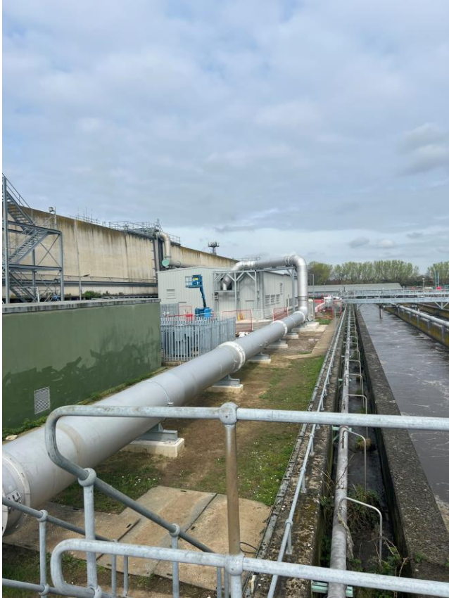
Battery D – new air main to ASP with connections
