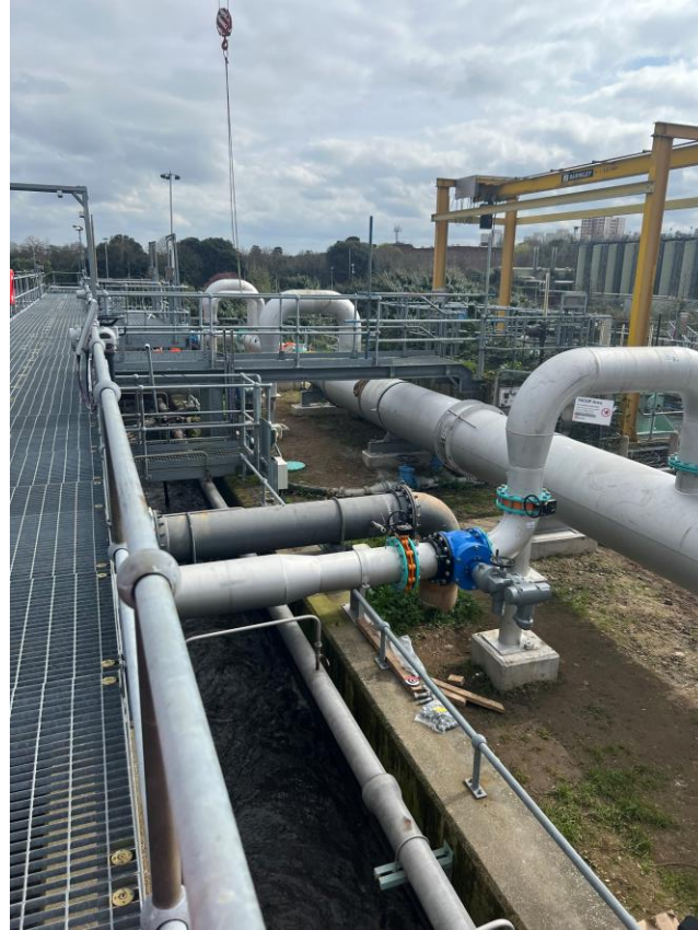
Battery D – new air main to ASP with connections
