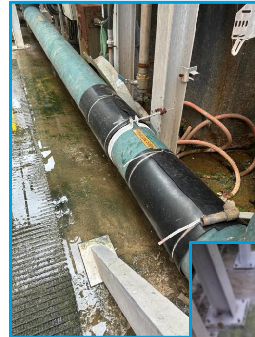
Collar-braced and cleaned OCU12 feed pipework
