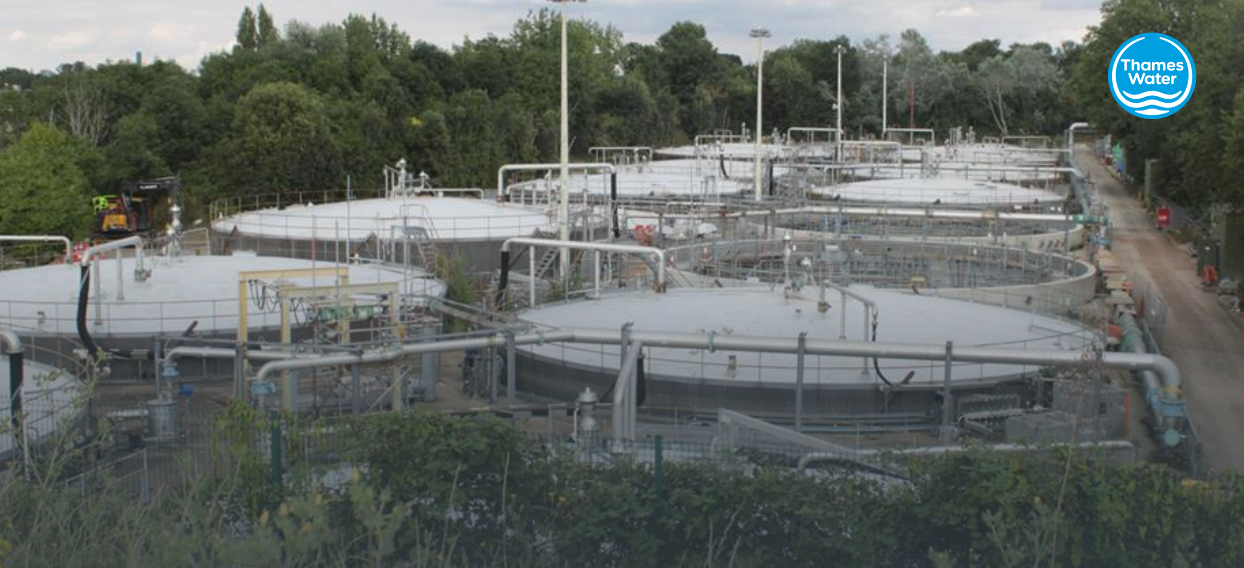
View of Digester Works
