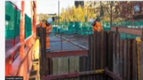
Works to replace Victorian pipes across the capital are under way
