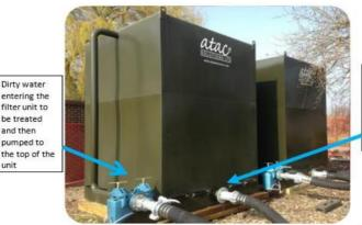
Treated water leaving the unit and returning to the environment
