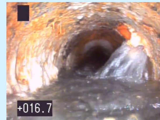
Figure 5: Infiltration gushing in around connecting pipe
