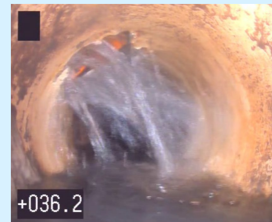
Figure 6: Infiltration gushing in around connecting pipe and past repair
