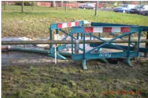
Photo 8 – Tankering used to pump out manhole (Buckskin).
