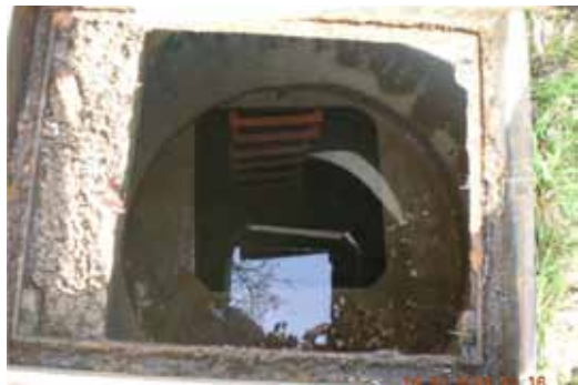
Photo 12 – Surcharged surface water manhole near old subway off Buckskin Lane (Buckskin).
