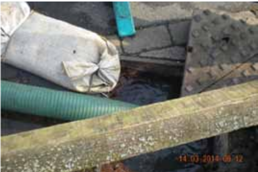
Photo 9 – Surcharged manhole (Buckskin).
