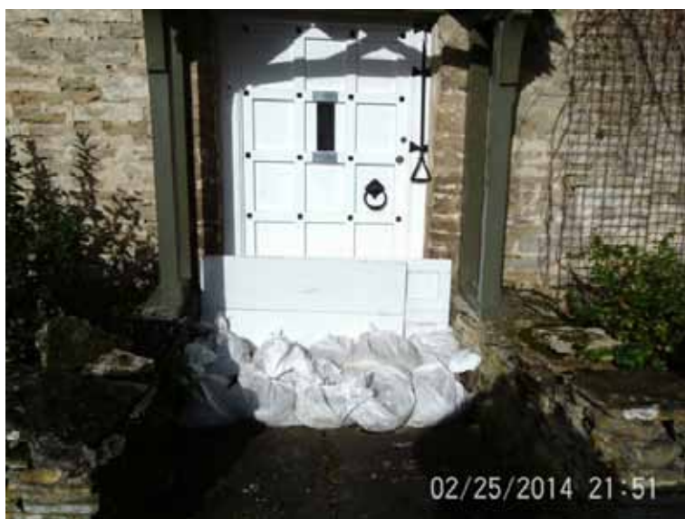
Photo 1 – Sandbags and flood boards to protect from river flooding in Shilton
