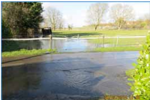
Photo 5 – Ditch north of village overflowing into fields and flowing into surface water drains on road
