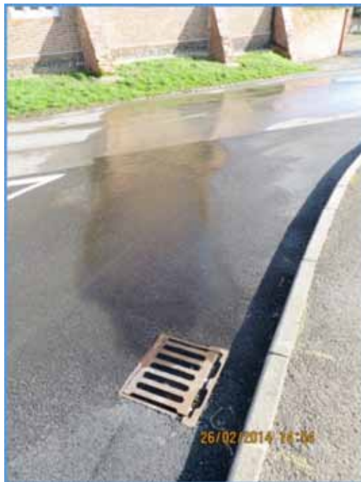
Photo 4 – Evidence of overflow from highway drain, Wallingford Road
