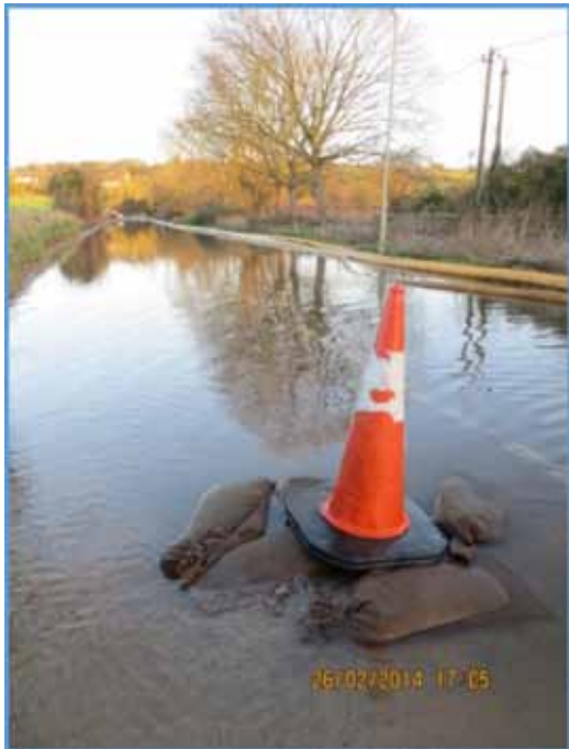
Photo 7 – Flooded Road and overflowing sewer – Aldworth Road
