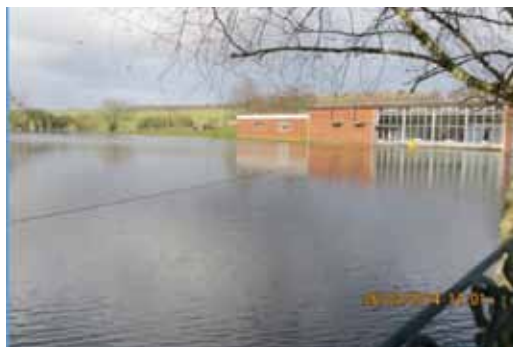
Photo 2 – Groundwater flooding in front of Compton Pumping station, Ilsley Road
