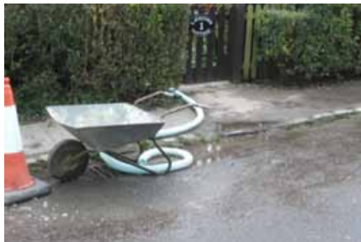
Photo 2 – Temporary pumping in Main Street.
