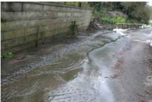
Photo 9 – Flooding in Upton.
