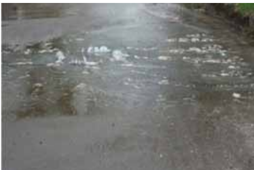
Photo 3 – Surcharged manhole in The Lane.
