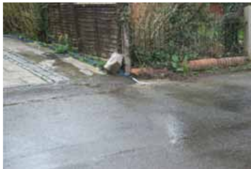
Photo 6 – Temporary pumping in Main Street.
