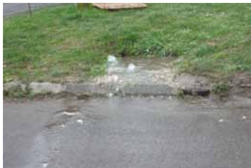
Photo 4 – Surcharged manhole.
