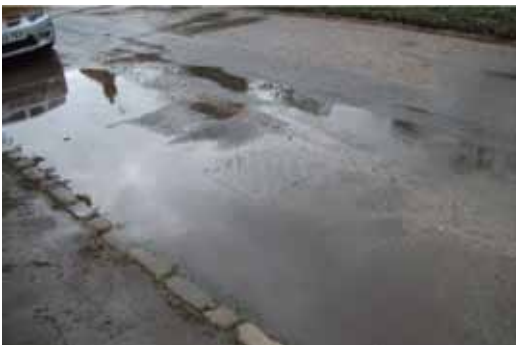
Photo 1 – Submerged manhole cover in Main Street.
