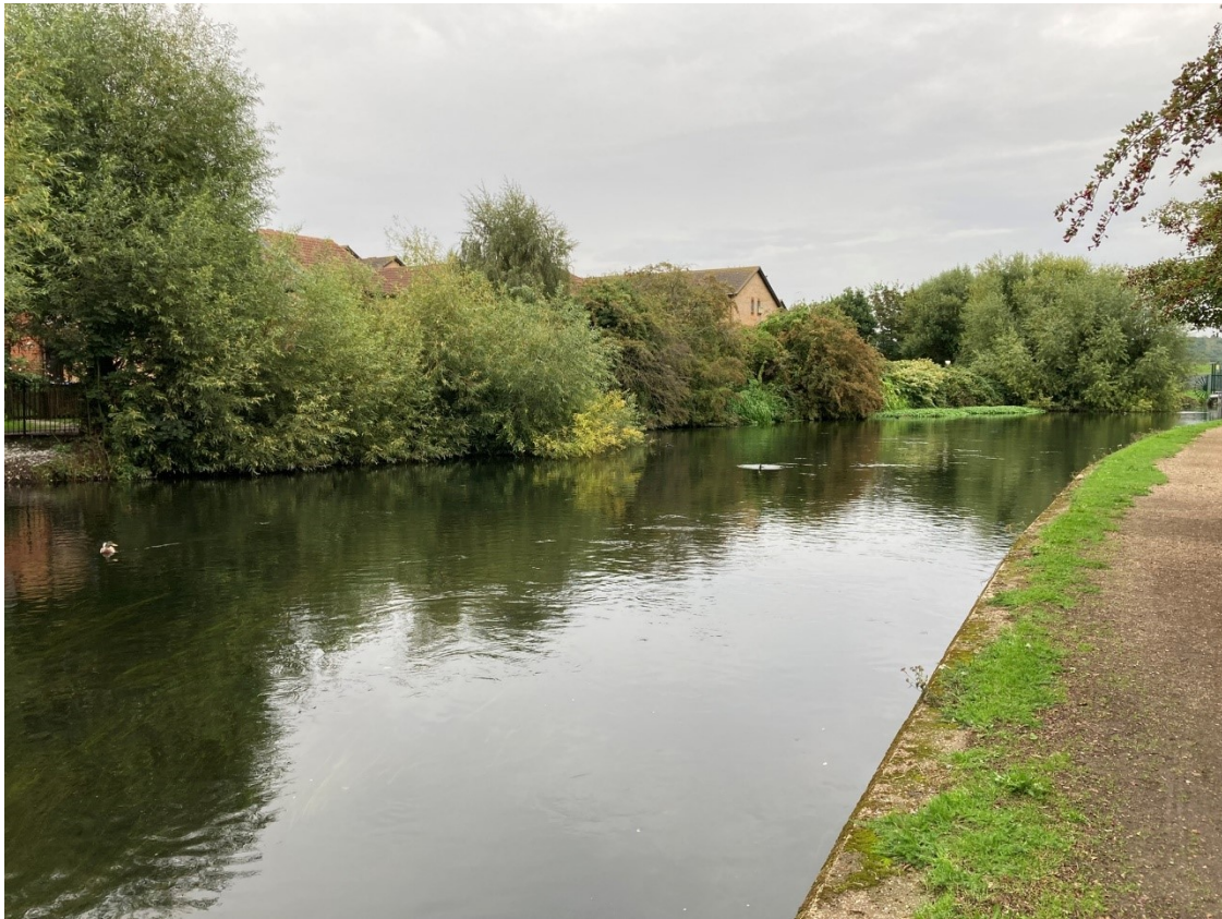
Figure 3-9 Enfield Island Loop of the Lee Diversion Channel from right bank looking downstream to the fenced area of the intake to King George V Reservoir
