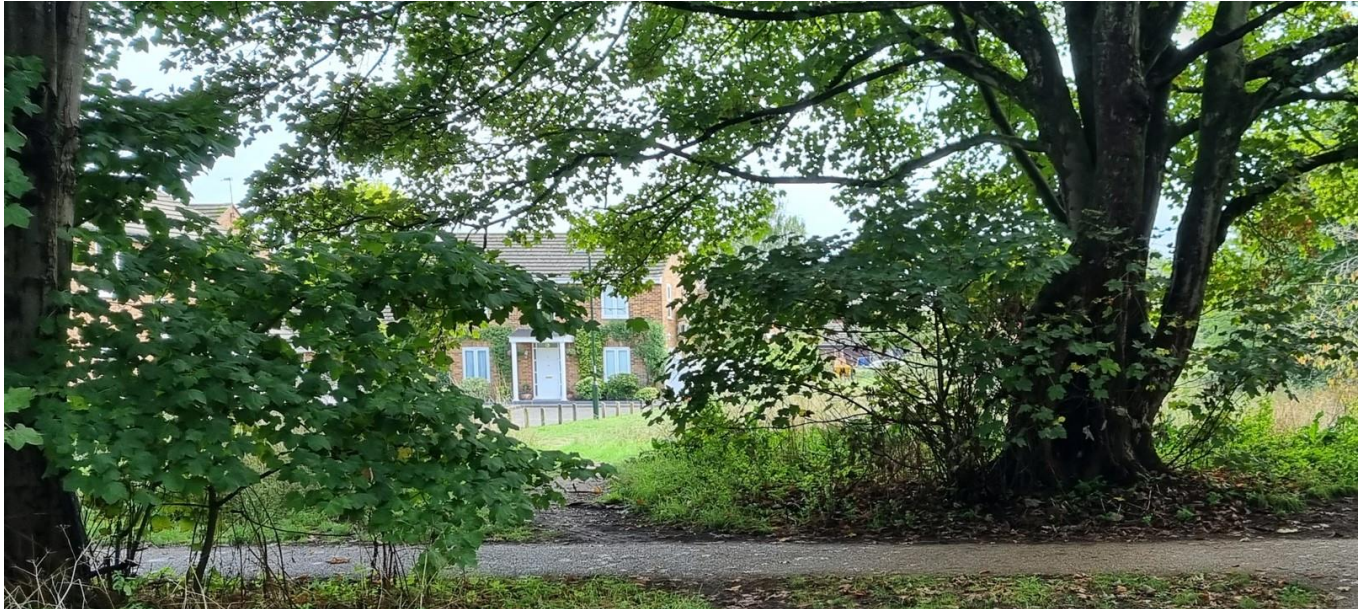
Figure 5: Typical site location for a pipe jacking chamber, in a nature reserve close to houses, on a small local street and adjacent to the River Thames
