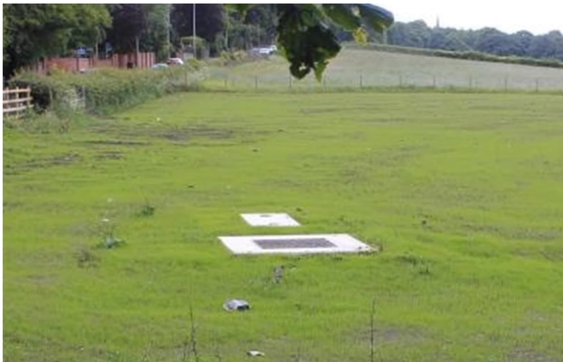
Figure 3.5 Typical Shaft Access Hatch after Completion
