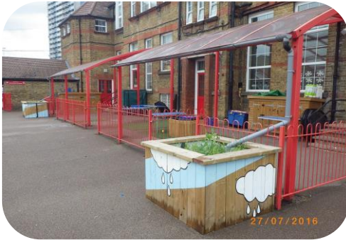
SuDS Rain planters at the end of downpipes
