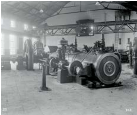
Littleton pumping station near view of engine, 1925
