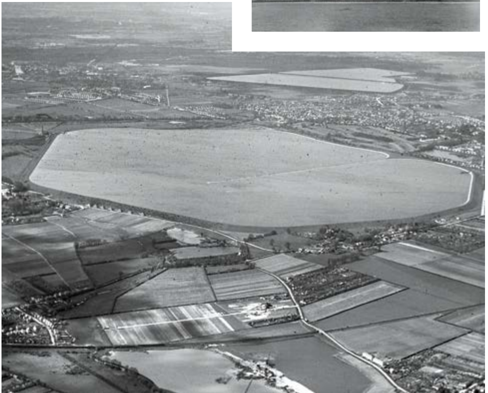
Above from top: Littleton pumping station’s group of European sanitary engineers, 1952; Aerial view of Queen Mary reservoir
