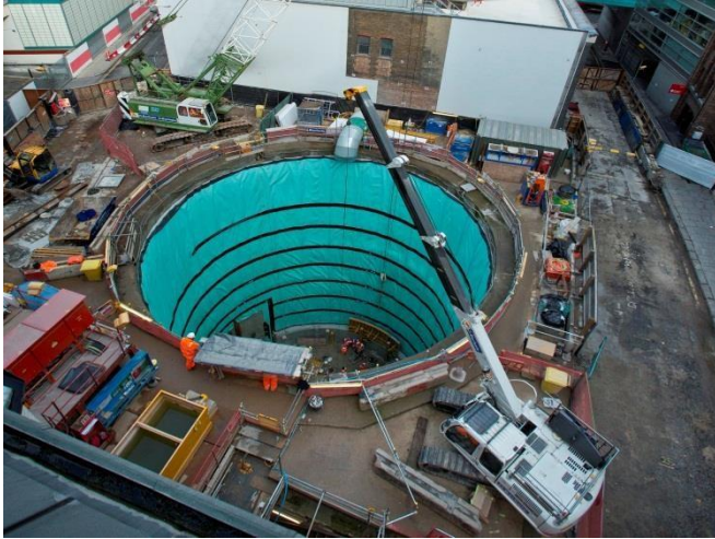
Deep excavation using heavy machinery
