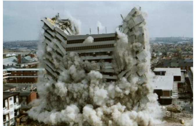
Demolition using explosives
