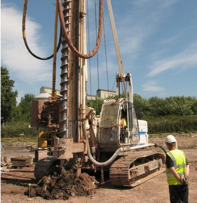
Continuous flight auger method of piling
