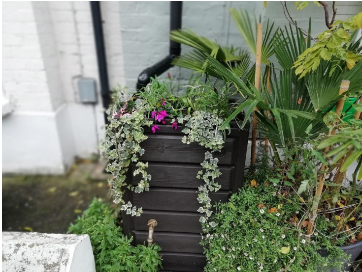
Figure 3 – Example of rainwater planter
