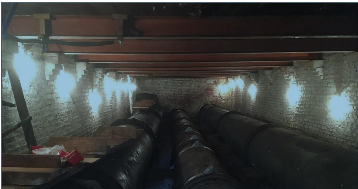
Figure 2: Open Culvert under [REDACTED]
